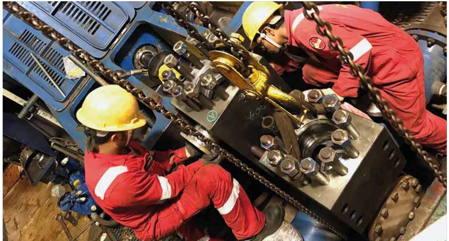
Mud pump reassembly.
