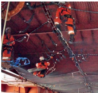
Temporary access platform – tensioned netting
