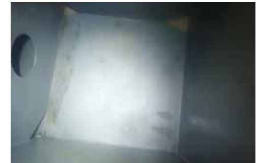
...and after cleaning.
