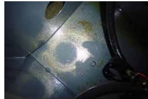
Drained reservoir before cleaning...
