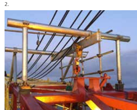
1. Frame assembled in workshop.
