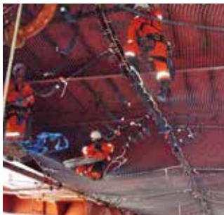
Temporary access platform – tensioned netting
