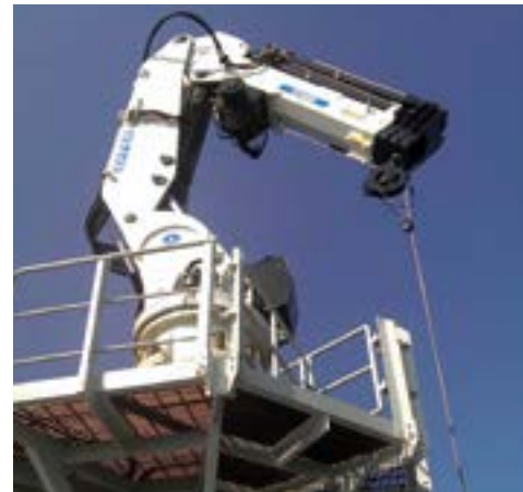
Fully functioning crane post- repair
